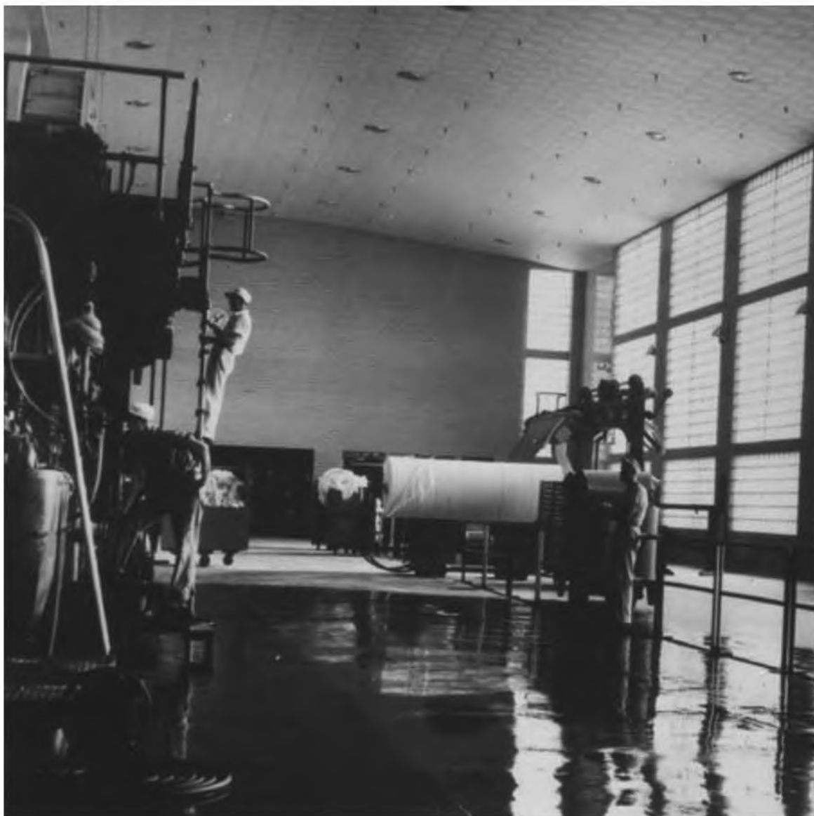
Kimberly Clark, Machine Building 3, Badger-Globe complex, Neenah, Wisconsin, 1940. Courtesy, Skidmore, Owings & Merrill
